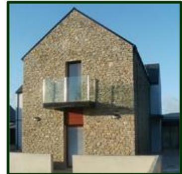
The old barn building had solid stone walls: to get the required U-value of  $0.26\text{W/m}^2\text{K}$ , a 75mm layer of Walltite was sprayed directly onto the interior wall surface, forming a seamless finish that is not only thermally efficient but is also airtight and watertight. The Walltite layer was then covered with plasterboard for the interior finish.
