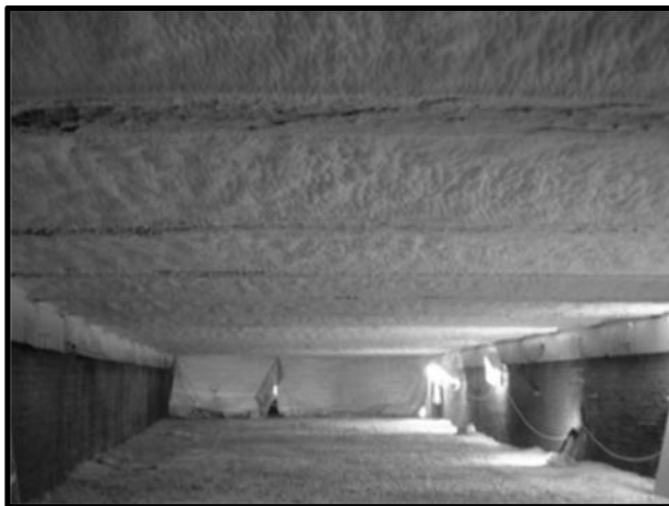
Figure 2: Bridge arch after stabilisation
