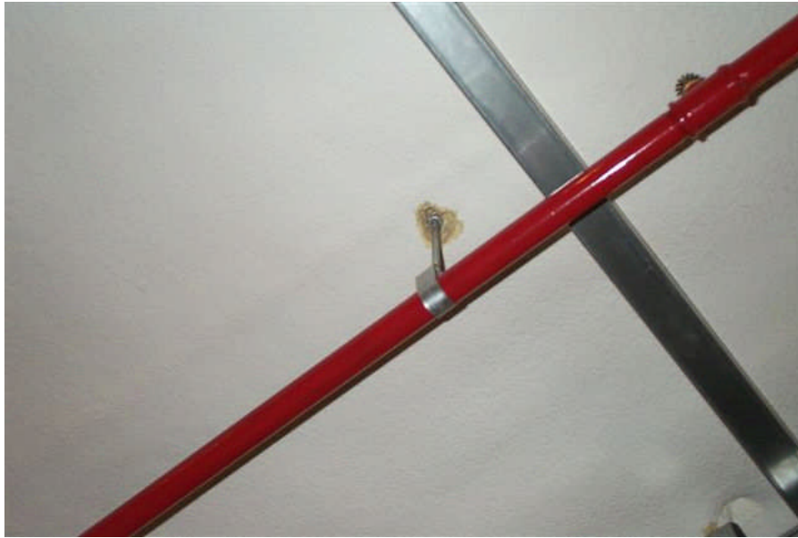
Picture shows: Polyurethane foam on ceiling close-up
