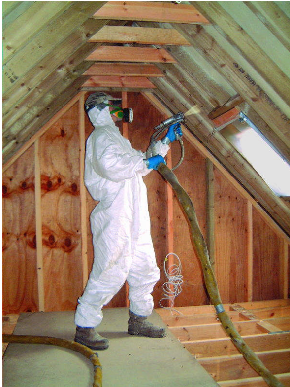
Picture shows: a BUFGA member spraying polyurethane foam.
